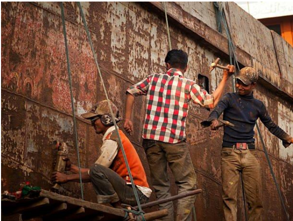
Ship repair workers on vessel hull — Sitakunda yard
